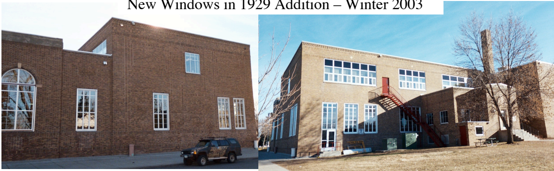
New Windows in 1929 Addition – Winter 2003
