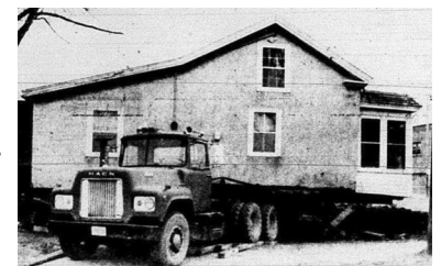
The tailor shop and home is being moved to The Landing.
