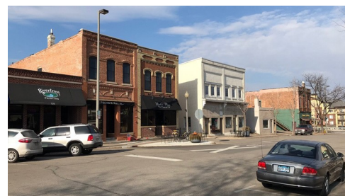
Part of the west side of Holmes Street in fall 2018
