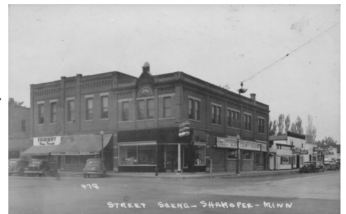
Looking southwest from the corner of Holmes Street and First Avenue in 1948
