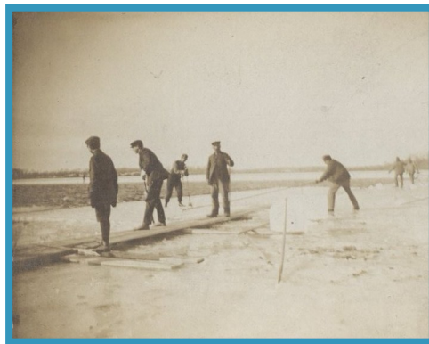
Ice harvesting on the Minnesota River at Shakopee. This photo shows a man holding a long wooden pole. Behind him is a wooden pulley system and conveyor belt used for moving blocks of ice.
