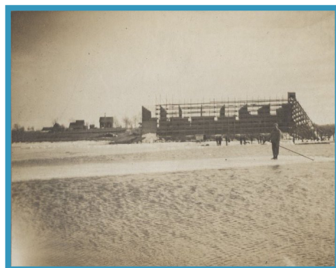
Workmen cutting ice on the Minnesota River at Shakopee. They are standing on a wooden boardwalk placed over the frozen river.
