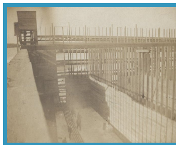
The front side of the wooden pulley system and conveyor belt. The wooden pulley system is constructed along the shore of the river. The front side shows areas divided by vertically placed pieces of wood. Blocks of ice available for purchase are stacked within each stall. The image is looking down into one stall, which contains blocks of ice, five workers and a wooden conveyor belt
