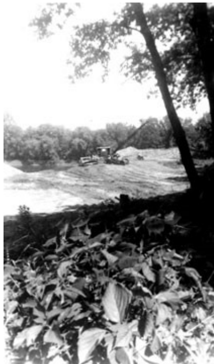
Excavating Cameron Marina, circa 1955.
