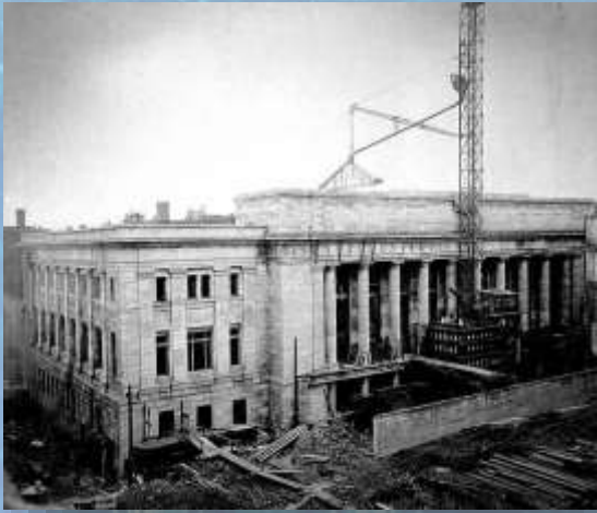
Under Construction c. 1921
